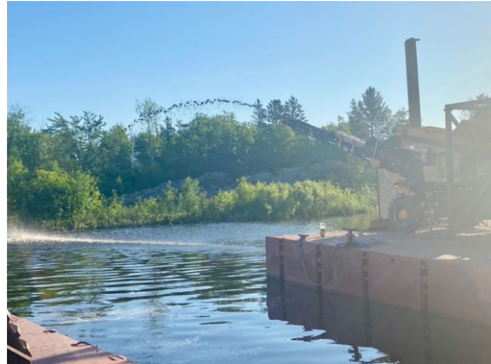
Slinger placing a proprietary PAC delivery technology (Source: Arcadis)
