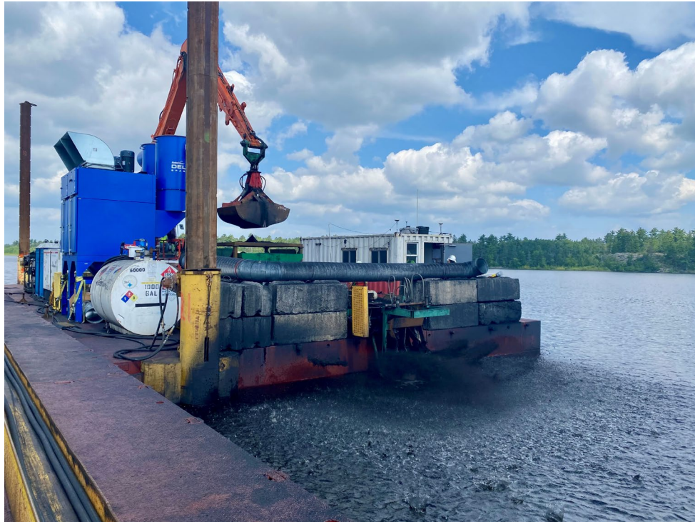
Proprietary placement method and PAC delivery technology (Source: Arcadis)
